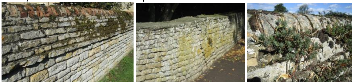
Variety of walls and appearance
