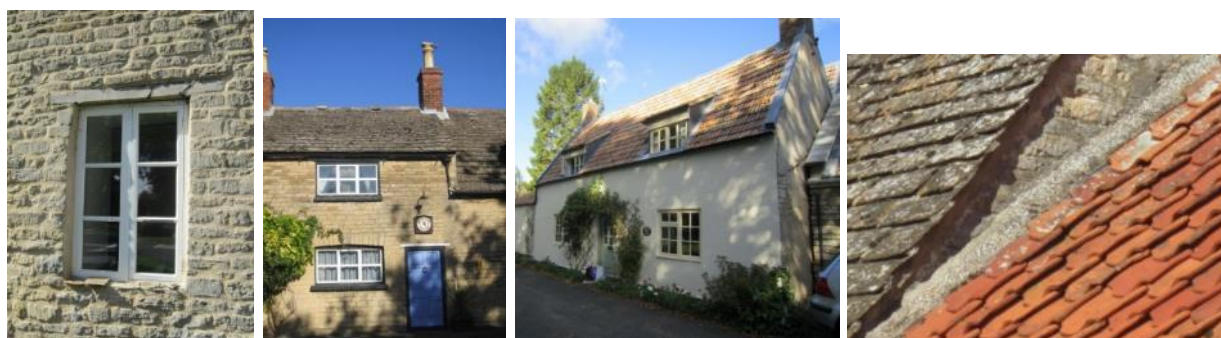
Limestone, Collyweston slate, triple roll pantile single lap pantile
