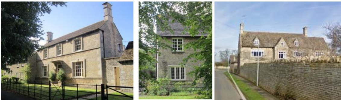
Limestone buildings with architectural dressings
